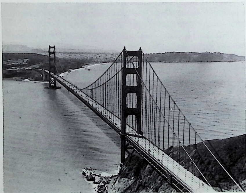
Above: a brick house shows compression strength; below: the Golden Gate Bridge in San Francisco is supported by a combination of compression and tension
