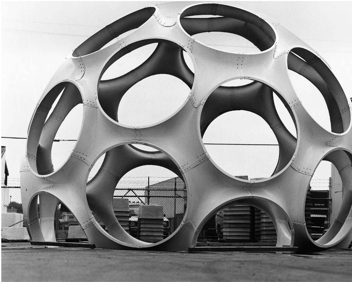
FIGURE 43. 50-foot-diameter Fly's Eye dome prototype
