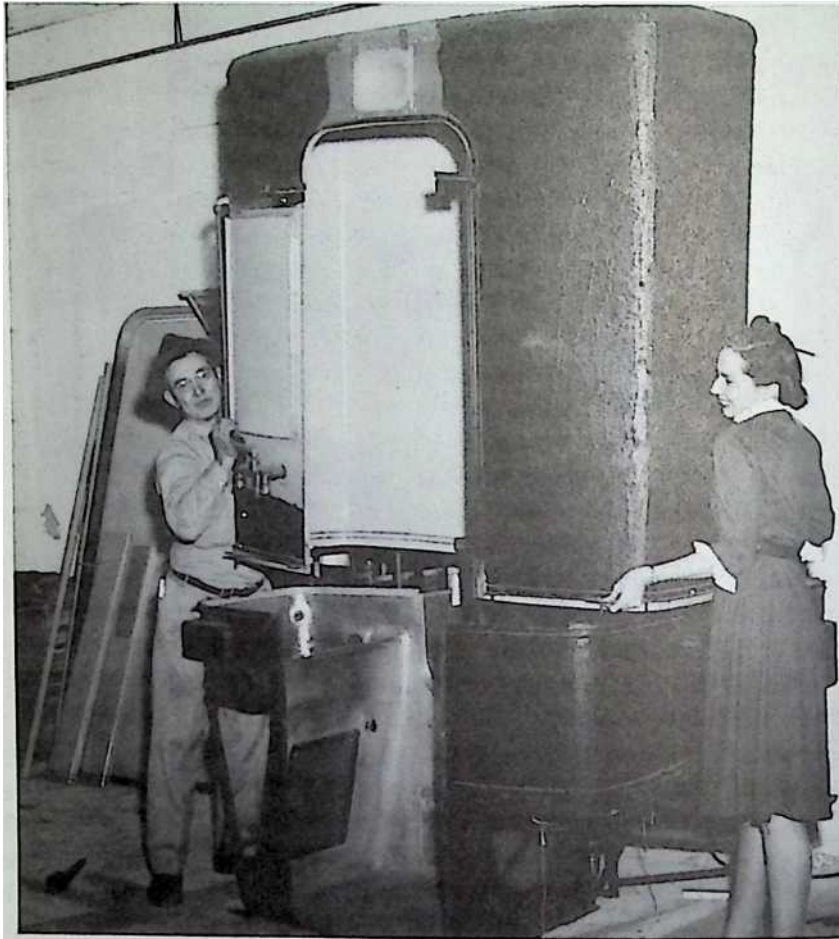
Fig. 9-3 The lightweight Dymaxion Bathroom sections being assembled.
