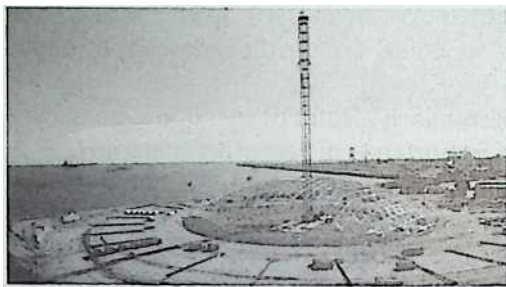
Fig. 15-6 The framework for the top is assembled around a central mast.
