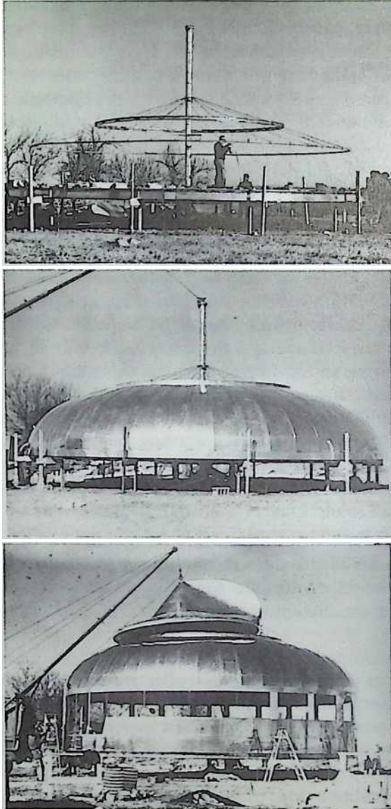
Fig. 12-1 through 12-3 Stages of erecting the Dymaxion House.
