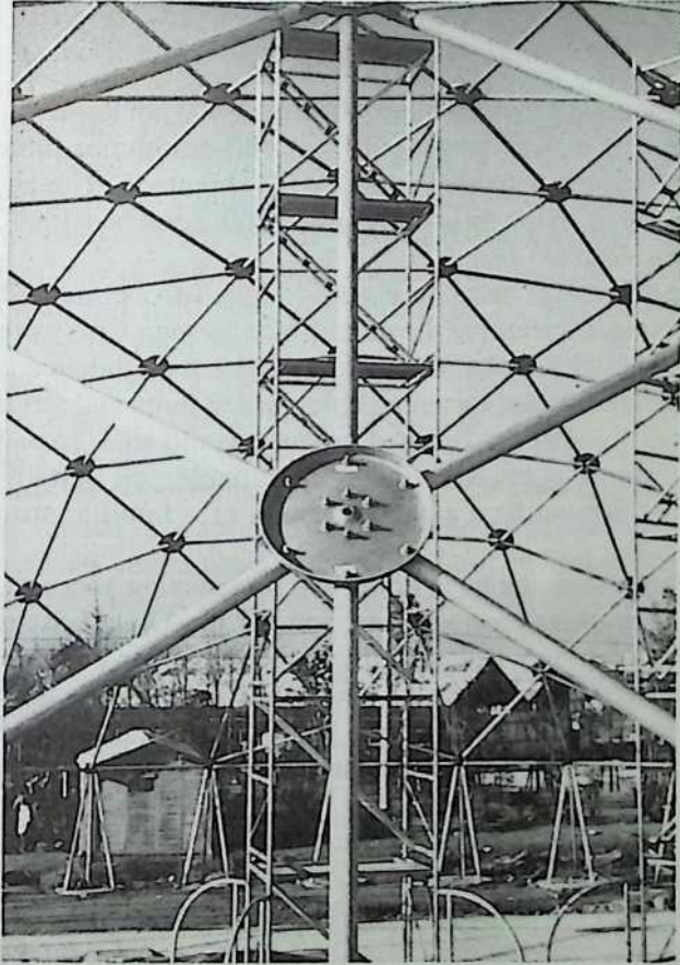
Fig. 14-1 The framework of the Afghan geodesic dome being erected.
