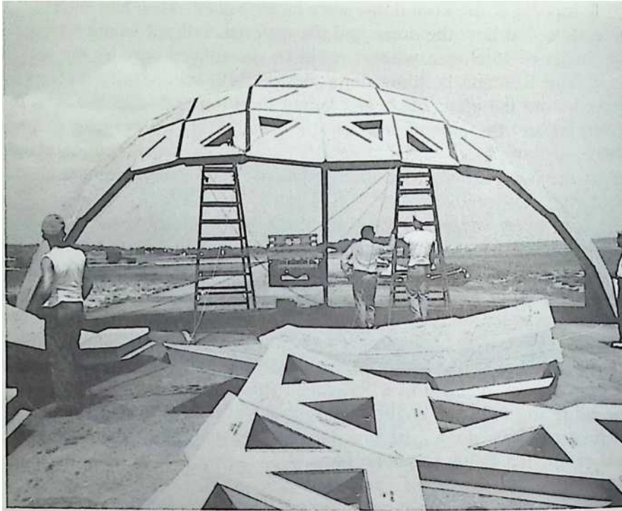
Fig. 14-9 A paperboard geodesic dome being erected.
